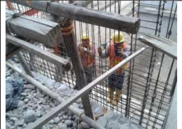
A photograph of a construction site showing the reinforcement of a concrete structure. A dense grid of steel bars is visible, with workers in safety gear working on it. The structure is supported by wooden beams and other construction elements.      |
